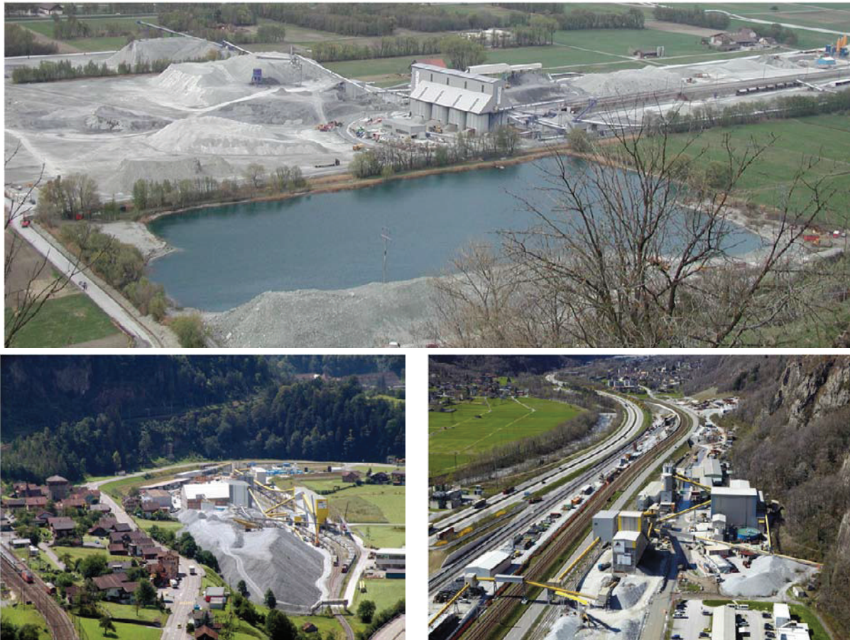
Figure 1. Spoil management sites with gravel plants AlpTransit. Above: Raron, Lötschberg base tunnel south; left: Amsteg, Gotthard base tunnel north (@ EBP AG); right: Bodio, Gotthard base tunnel south (@ AlpTransit Gotthard AG)
